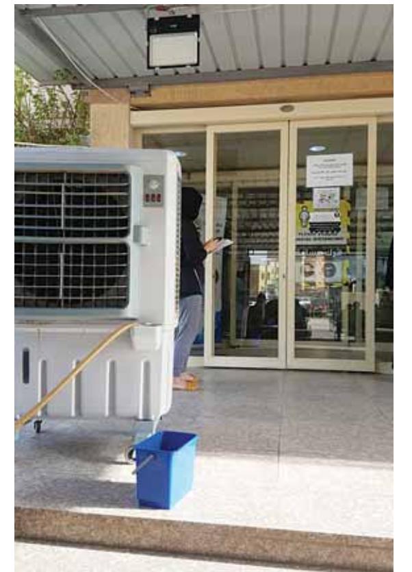
KUWAIT: Patients visiting the West Salmiya Policlinic are seated outside the building waiting in the heat for their turn to get to see the doctor. An AC unit is placed at the outdoor waiting area, although patients have complained that it was not working or "making any difference" under the extreme heat.
