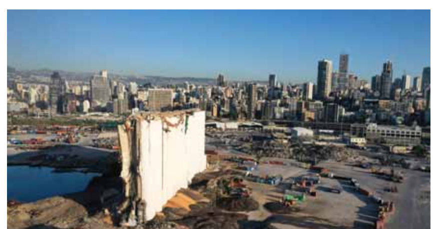
BEIRUT: An aerial view shows Beirut port on May 27, 2021, damaged in a massive explosion on Aug 4 last year, which killed more than 200 people and injured scores of others. — AFP
