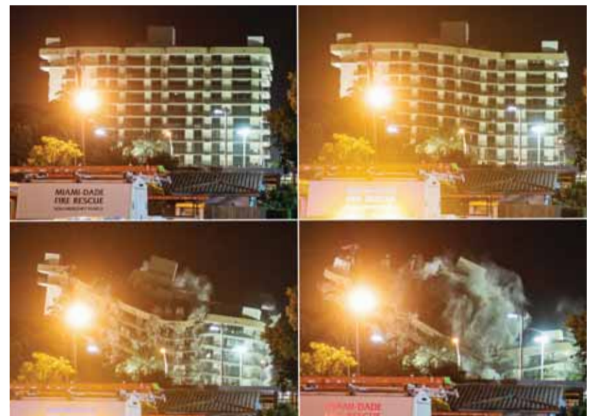
SURFSIDE, Florida: This combination of pictures created on July 4, 2021 shows the rest of the Champlain South tower just before being demolished (top L) and as it is demolished by a controlled explosion in Surfside. —AFP
