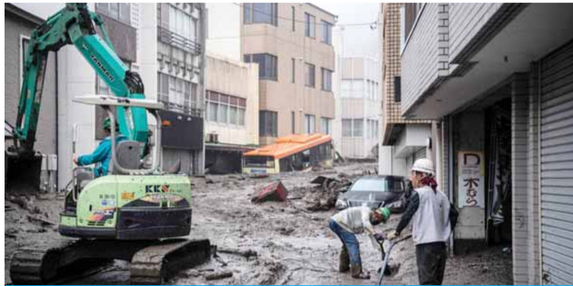
ATAMI: Workers remove mud and debris at the scene of a landslide following days of heavy rain in Shizuoka Prefecture yesterday. — AFP
