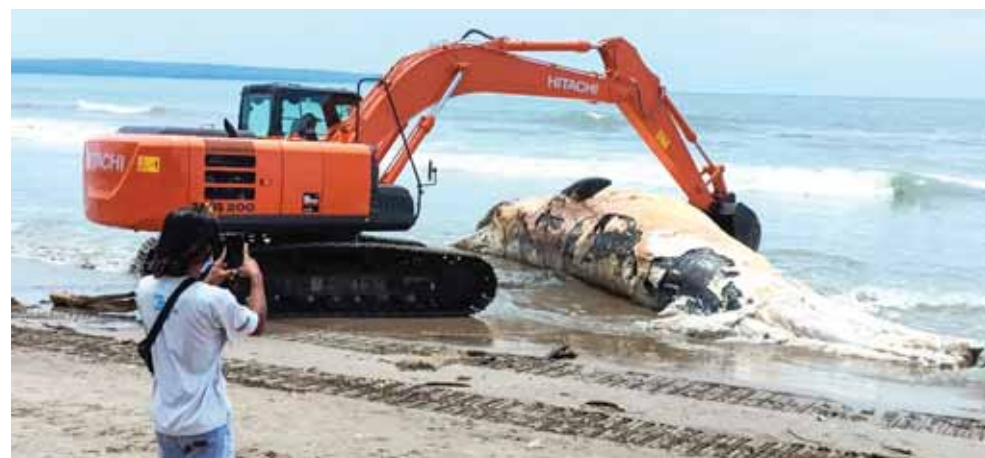
This handout photo shows workers on an excavator preparing to bury the carcass of a giant 13-metre whale washed up on Batu Belig beach, on Indonesia’s holiday island of Bali.
