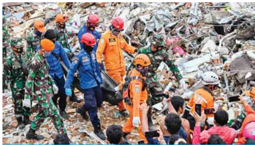
MAMUJU: Rescuers move the body of a victim that was trapped in a collapsed building in Mamuju yesterday. — AFP
