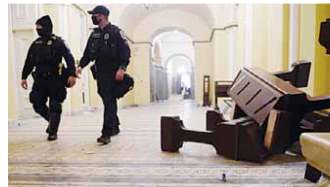
WASHINGTON, DC: Damage is seen inside the US Capitol building early yesterday in Washington, DC, after supporters of US President Donald Trump breached security and entered the building during a session of Congress. —AFP
