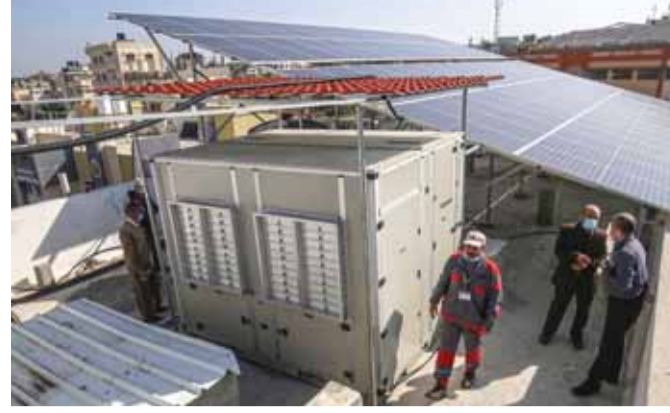
A picture shows a solar-powered water generator that extracts potable water straight from the air donated by Watergen in the Palestinian town of Khan Yunis in southern Gaza Strip. — AFP photos
