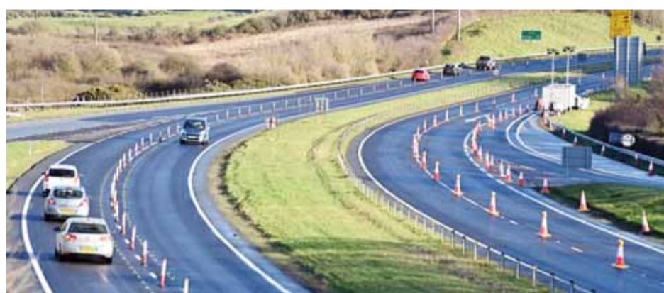
Cars travel through a contraflow system on the westbound A55 in Anglesey in north Wales on January 02, 2021. The carriageway is closed to traffic to create queuing areas for vehicles travelling into Holyhead port and on to Dublin in Ireland. —AFP
