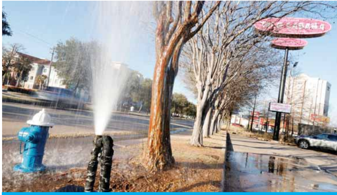
HOUSTON, Texas: Water shoots out of a burst pipe outside of a restaurant on Saturday in Houston, Texas. Much of Texas is still struggling with historic cold weather, power outages and a shortage of potable water after winter storm Uri swept across 26 states with a mix of freezing temperatures and precipitation. — AFP
