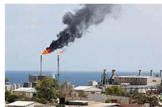
A general view of the Zawiyah oil installation in Libya in this file photo. — AFP
