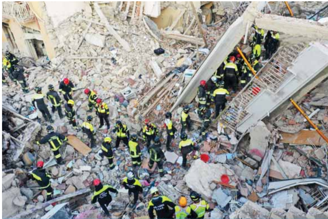
RAVANUSA: This handout picture taken and released by Italian Firefighters (Vigili del Fuoco) shows a four-storey apartment building collapsed, following a gas explosion, in Ravanusa on December 12, 2021. — AFP
