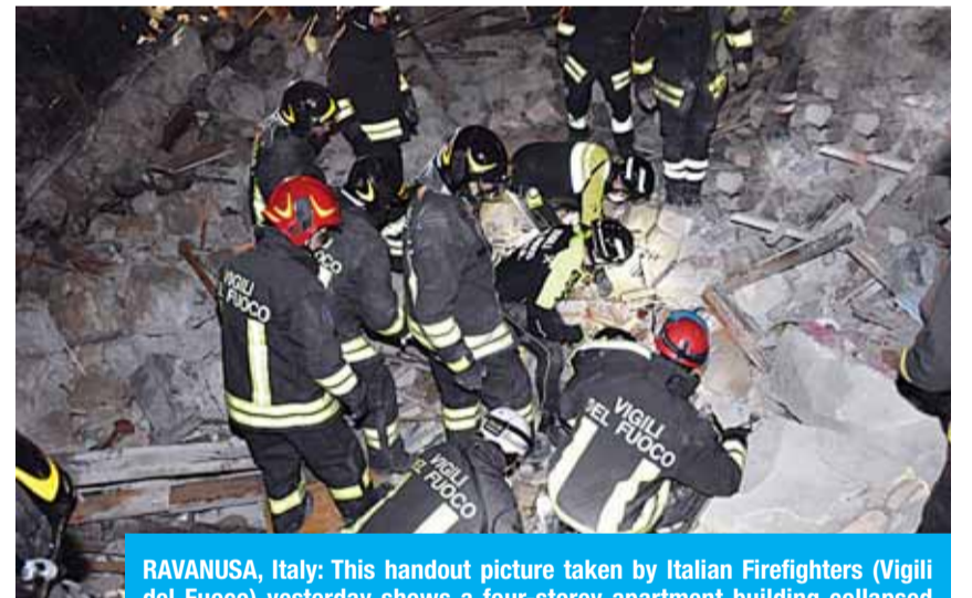
RAVANUSA, Italy: This handout picture taken by Italian Firefighters (Vigili del Fuoco) yesterday shows a four-storey apartment building collapsed following a gas explosion, in Ravanusa yesterday. —AFP
