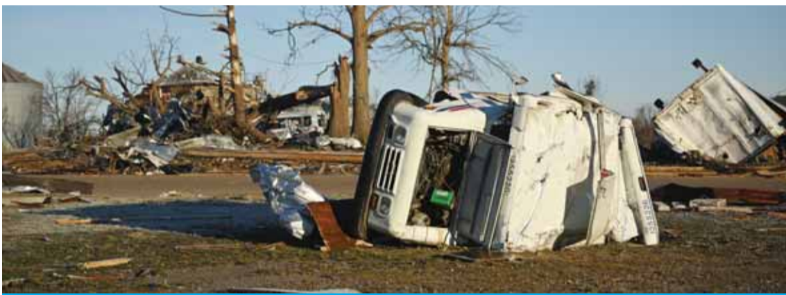
MAYFIELD: Tornado damage is seen yesterday after extreme weather hit the region in Mayfield, Kentucky. — AFP
