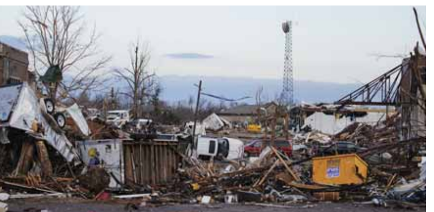
MAYFIELD, Kentucky: Heavy damage is seen downtown after a tornado swept through the area yesterday. — AFP
