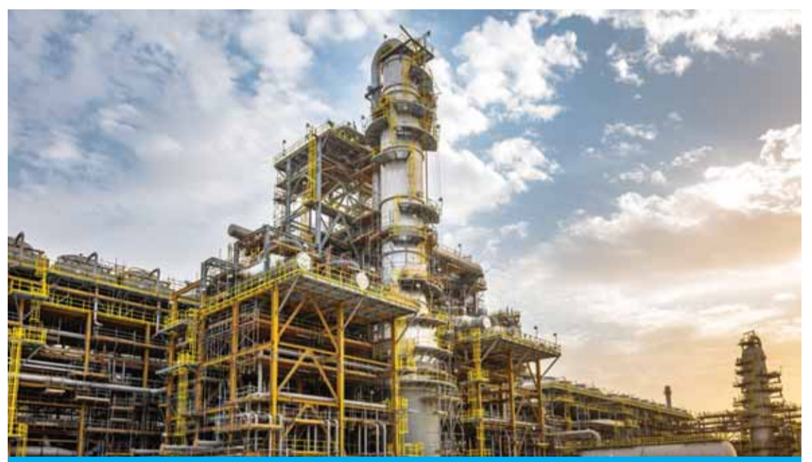
JUBAIL, Saudi Arabia: Saudi Aramco's Fadhili Gas Plant Project, located 30 km west of the city of Jubail in the eastern province of Saudi Arabia. —AFP
