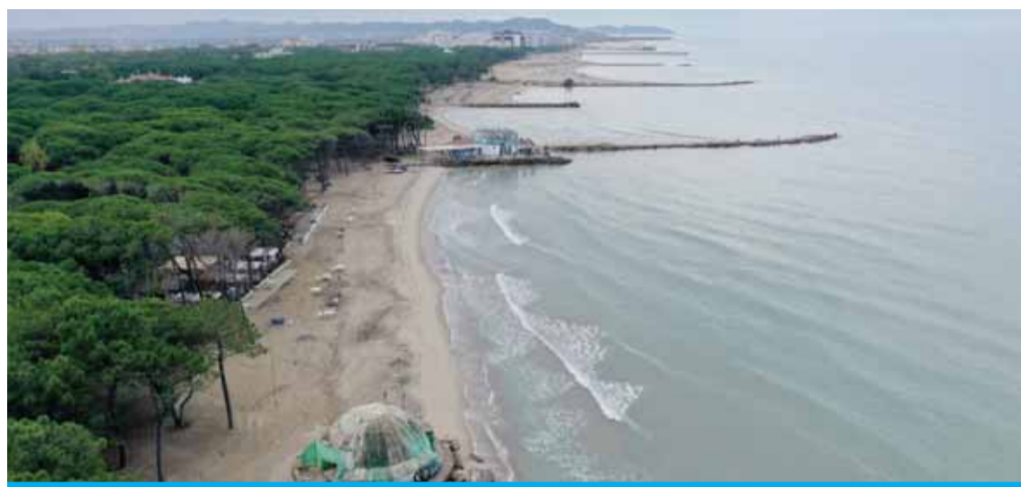
KAVAJE, Albania: This photograph taken in Qerret shows an aerial view of a communist-era bunker (front) and the groynes built on the Adriatic shore. —AFP
