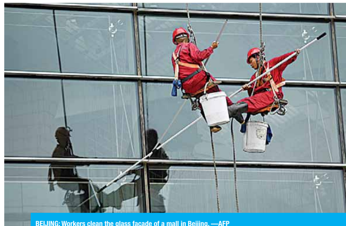
BEIJING: Workers clean the glass facade of a mall in Beijing. —AFP
