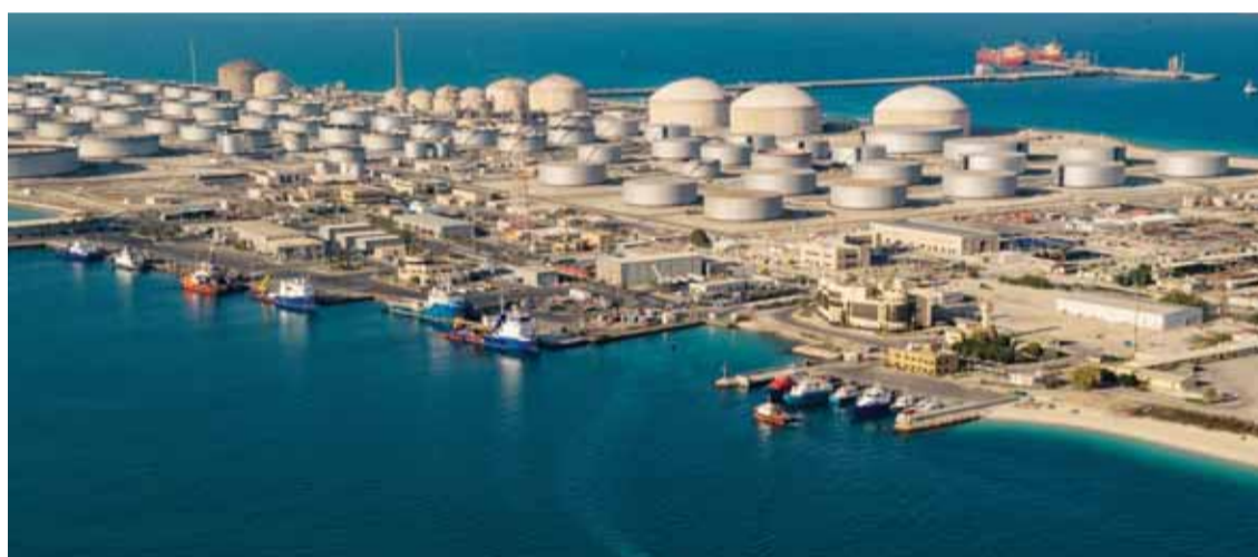
DHAHRAN: File handout picture shows Saudi Arabia's state-owned oil and gas company's Dhahran oil plants, in eastern Saudi Arabia. Aramco said yesterday its second quarter profits for 2021 nearly quadrupled compared to the same period last year. — AFP
