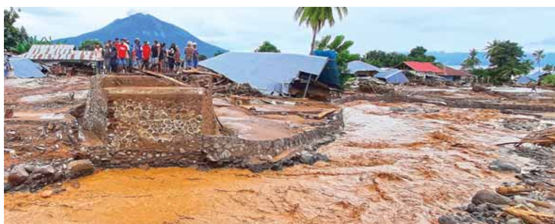
Damaged homes after a flash flood in Waiwerang village, East Flores. At least 157 people have been killed in Indonesia and neighboring East Timor with dozens more still missing after a tropical cyclone battered the Southeast Asian nations. — AFP
