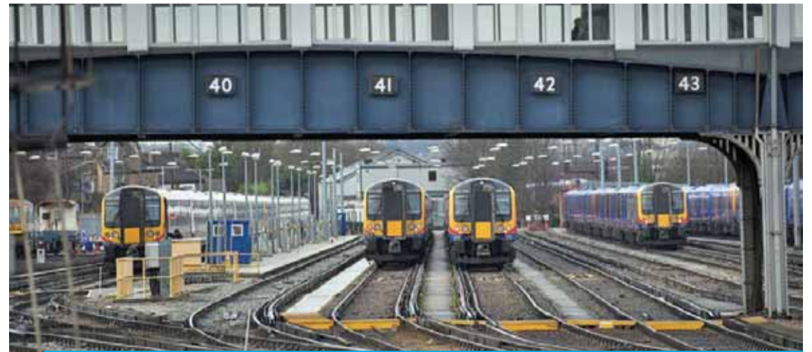
LONDON: Trains are seen at Clapham Junction train station in south London. Britain unveiled on Monday a radical overhaul of its coronavirus-plagued privatized rail sector that will see franchises replaced with concessions subject to tougher scrutiny and greater state involvement. — AFP
