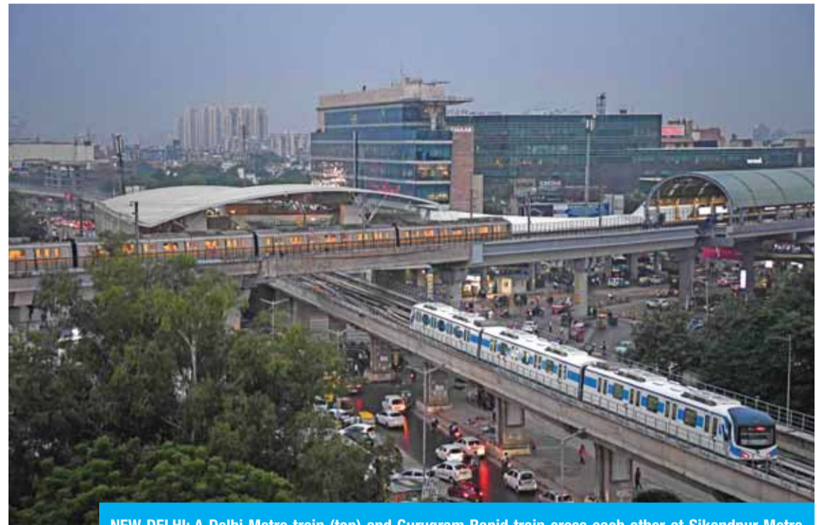
NEW DELHI: A Delhi Metro train (top) and Gurugram Rapid train cross each other at Sikandpur Metro station as Delhi Metro Rail Corporation (DMRC) resumed its services on Yellow line from Samaypur Badli to Huda city centre in Gurugram. — AFP
