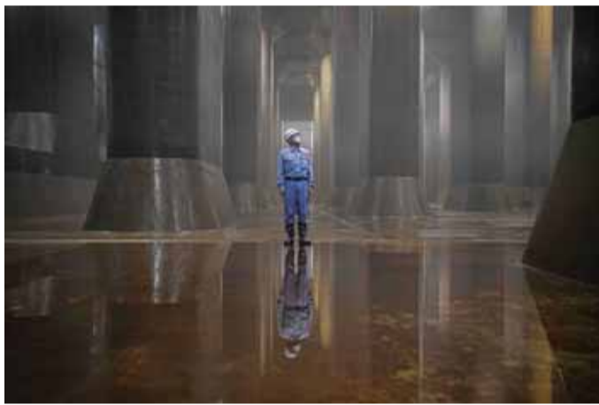
In this photo an employee stands in the water tank of the metropolitan outer underground discharge channel in Kasukabe, Saitama prefecture.
