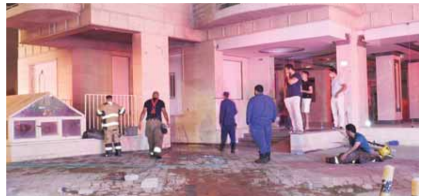
KUWAIT: Firefighters seen outside a Mangaf building where a blaze was reported.
