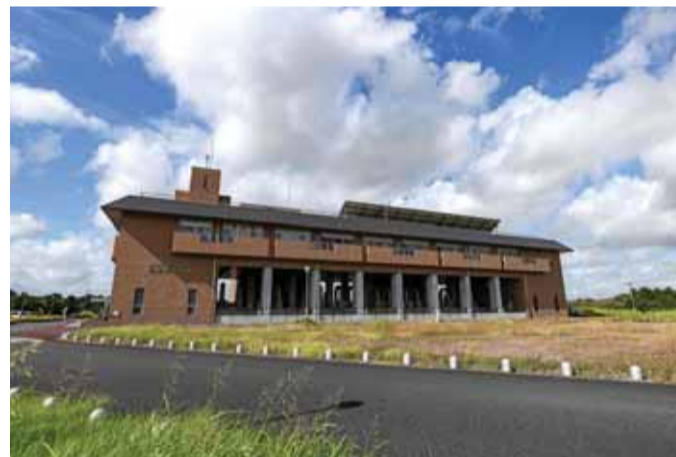
The main building of the metropolitan outer underground discharge channel is pictured in Kasukabe, Saitama prefecture.
