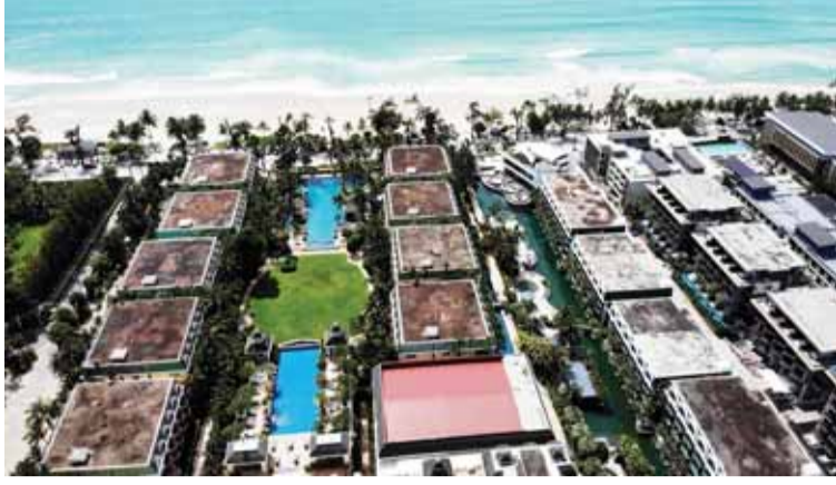
This aerial photo shows empty swimming pools in a row of hotels on Patong beach in Phuket.
