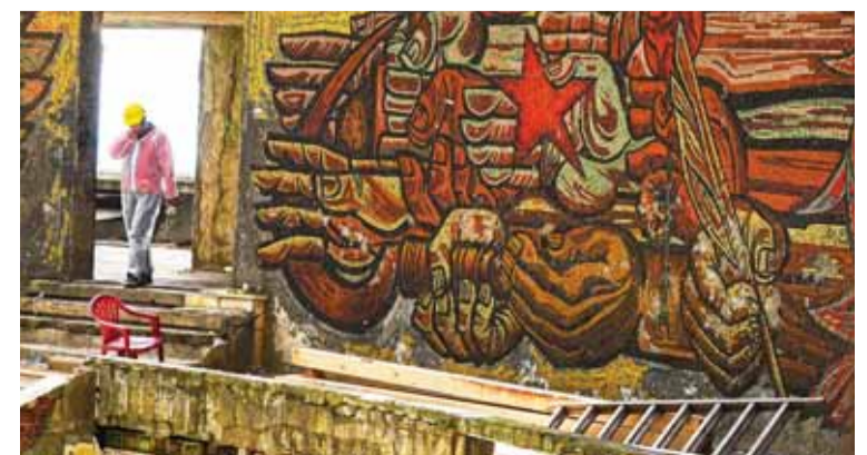
A construction expert walks near a mosaic inside the House of the Bulgarian Communist Party.
