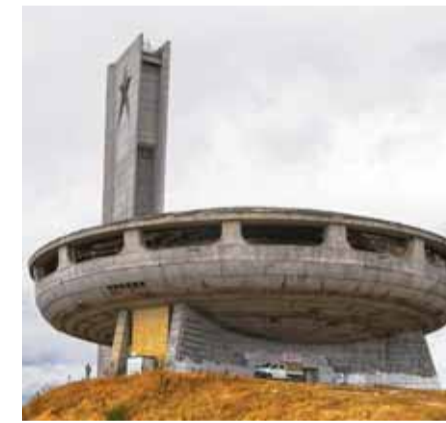
A picture shows the House of the Bulgarian Communist Party on Buzludzha peak in central Bulgaria.
