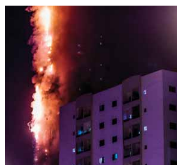
SHARJAH: People stand on a bridge and watch a fire that erupted in a 48-storey residential tower on Tuesday. — AFP
