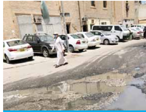
Overflowing sewage in Hasawi.
