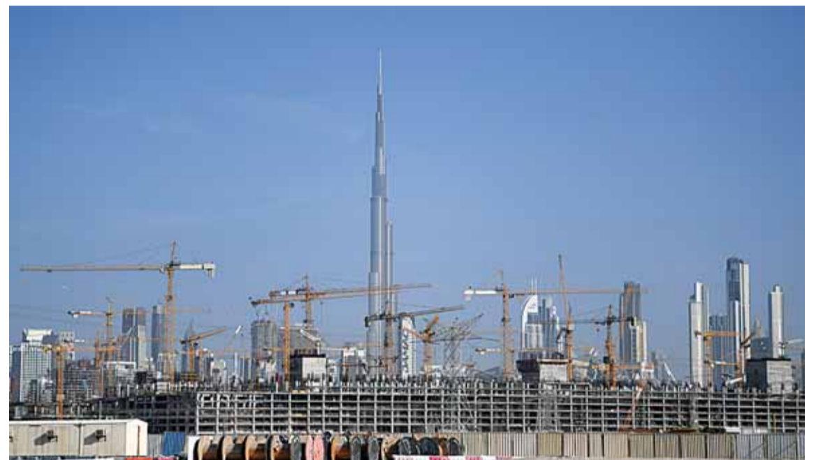
DUBAI: A general view of construction projects in Dubai that require a big number of workers and are currently empty due to fears of the spread of the coronavirus in the Gulf emirate yesterday. —AFP
