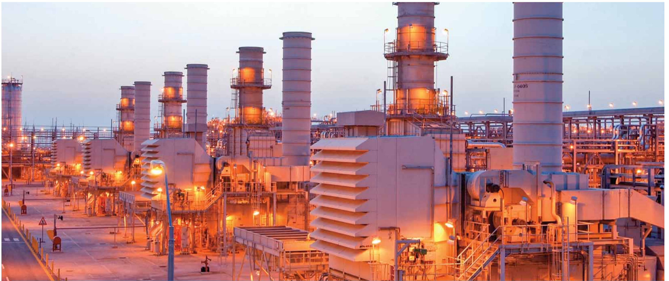
Energy giant Saudi Aramco shows its gas facilities at Yanbu refinery. On top of war and the coronavirus pandemic, Yemen faces looming economic disaster as a crisis gripping its main benefactor Saudi Arabia dents remittances and leaves state coffers running dry. — AFP
