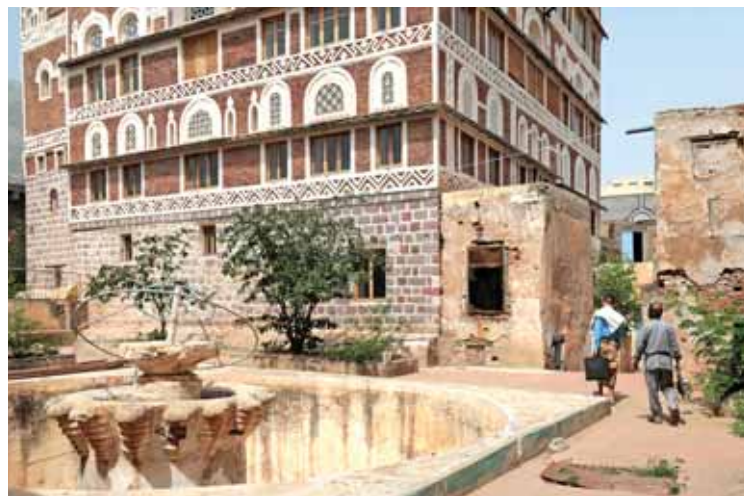
A picture shows a facade, that has been restored, at the National Museum in Yemen's third city of Ta'ez.
