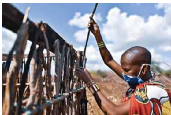
A woman from the Maasai tribe constructs a wall by twining sticks around a wooden structure of a traditional shelter at their manyatta (village) in Talek.
