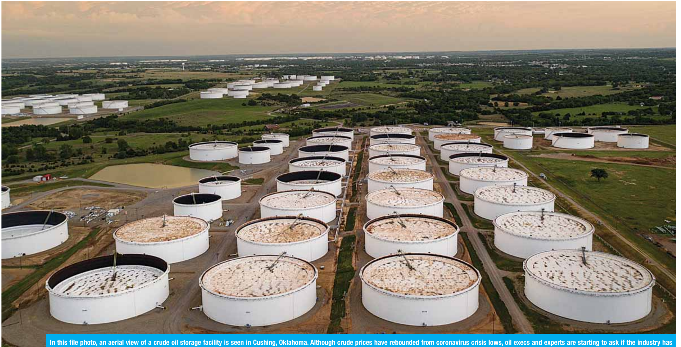
In this file photo, an aerial view of a crude oil storage facility is seen in Cushing, Oklahoma. Although crude prices have rebounded from coronavirus crisis lows, oil execs and experts are starting to ask if the industry has crossed the Rubicon of peak demand. —AFP
