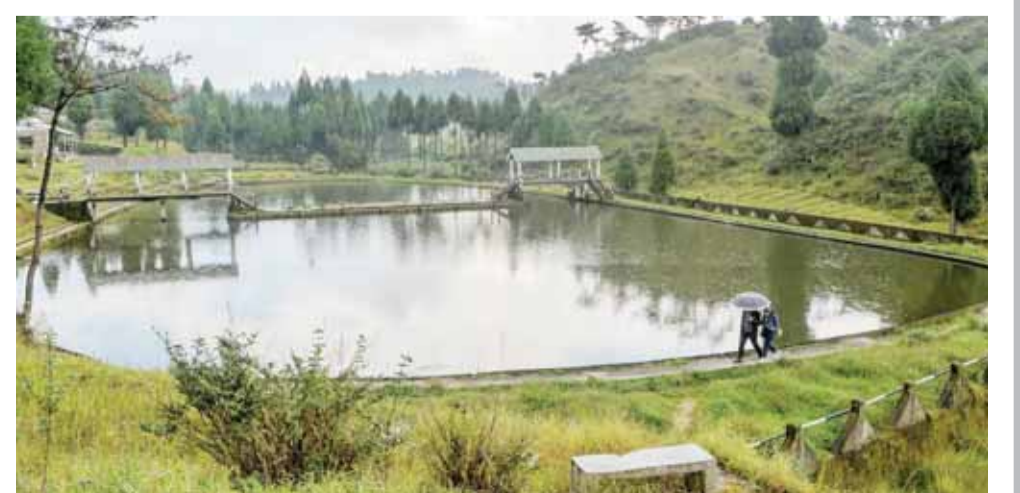
This picture taken on Sept 19, 2019 shows a general view of the water harvesting pond and drainage retaining wall at Nongthymmai-Lumthangding village on the outskirts of Shillong in Meghalaya.
