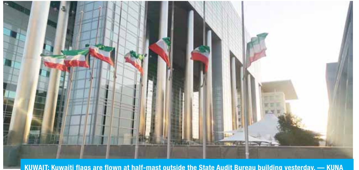
KUWAIT: Kuwaiti flags are flown at half-mast outside the State Audit Bureau building yesterday. — KUNA
