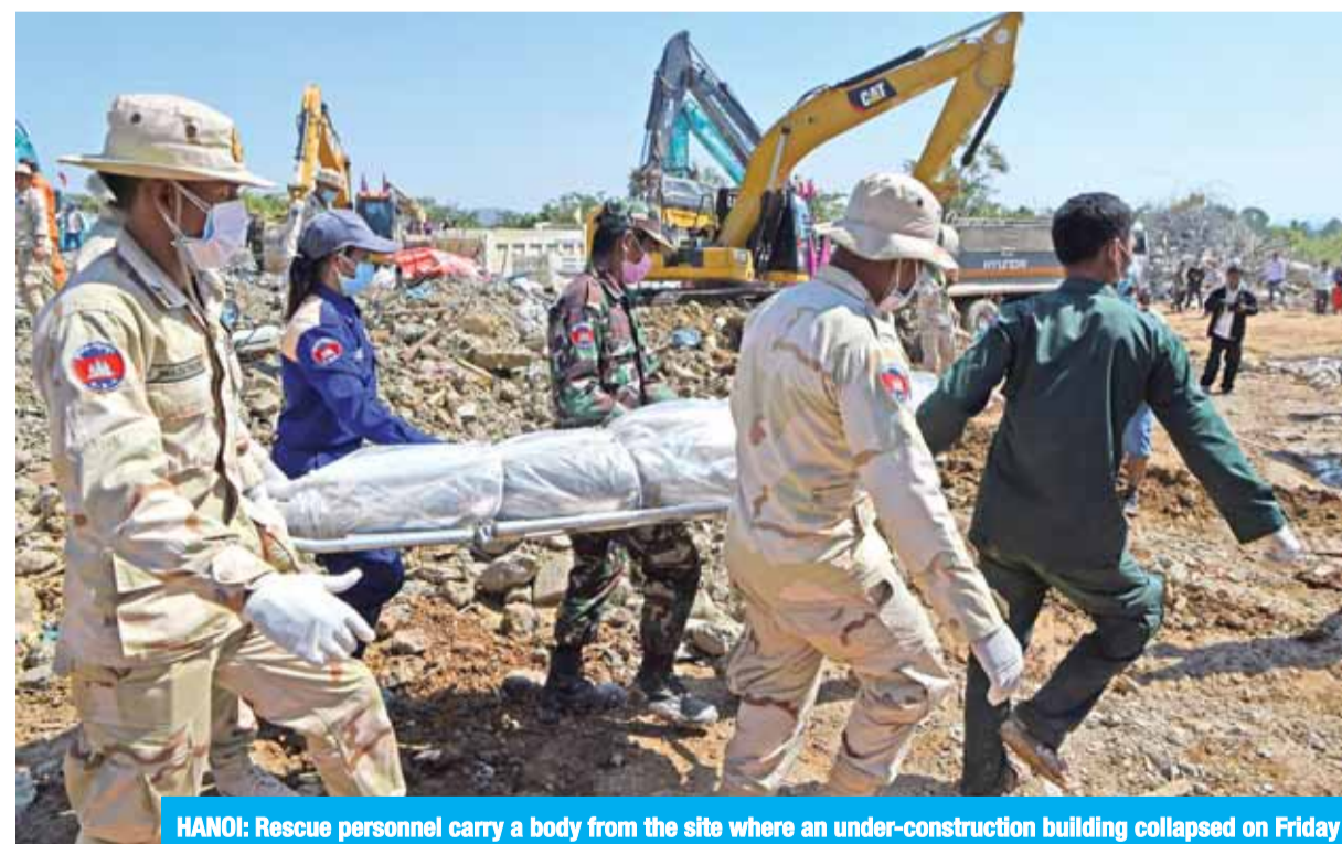
HANOI: Rescue personnel carry a body from the site where an under-construction building collapsed on Friday in southern Cambodia's coastal Kep province yesterday. — AFP
