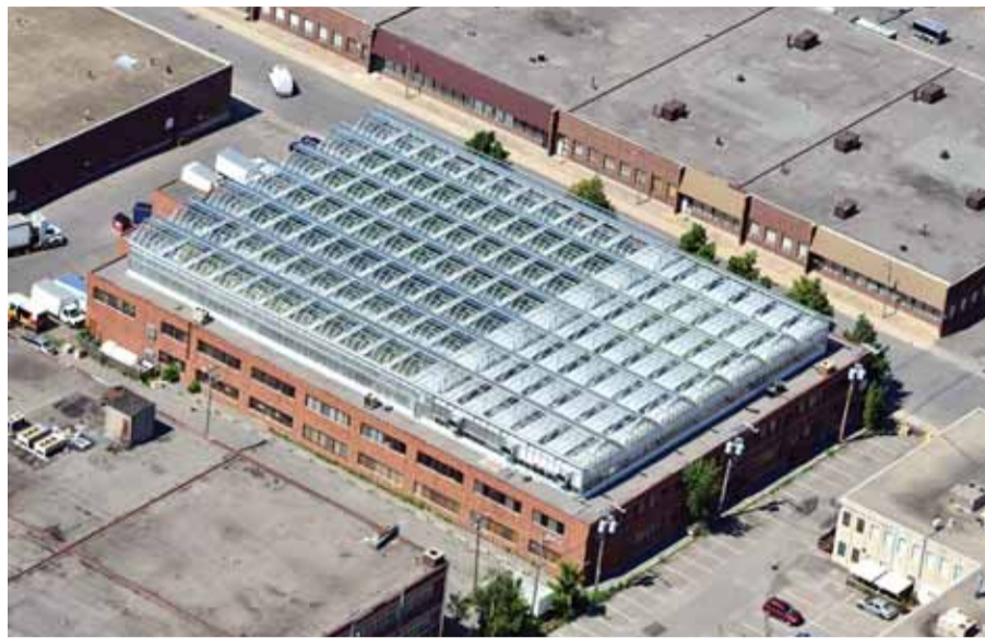
Lufa Farms just opened what it says is the world's largest commercial rooftop greenhouse, seen in this aerial photo in Montreal.
