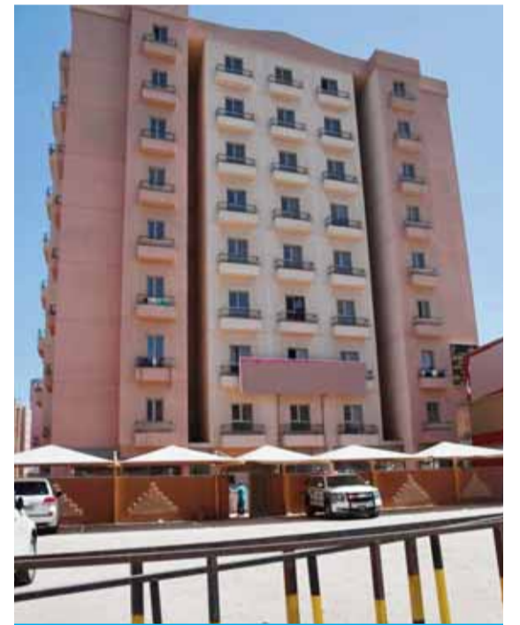
KUWAIT: A building in Mahboula is under lockdown after the discovery of three cases of coronavirus among Asian workers residing there. — Photo by Fouad Al-Shaikh
