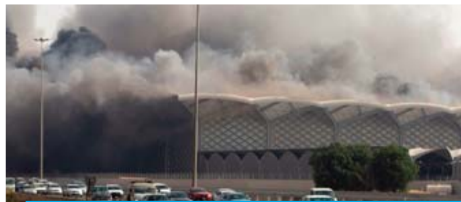
JEDDAH: Cars drive by as thick smoke billows from the Haramain high-speed train station after a fire broke out yesterday. — AFP
