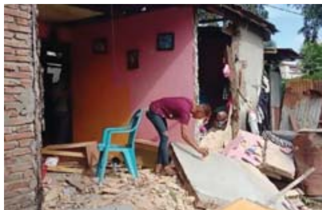
AMBON CITY: A resident inspects a collapsed wall of his house in Ambon, Indonesia's Maluku islands following a 6.5-magnitude earthquake yesterday. — AFP
