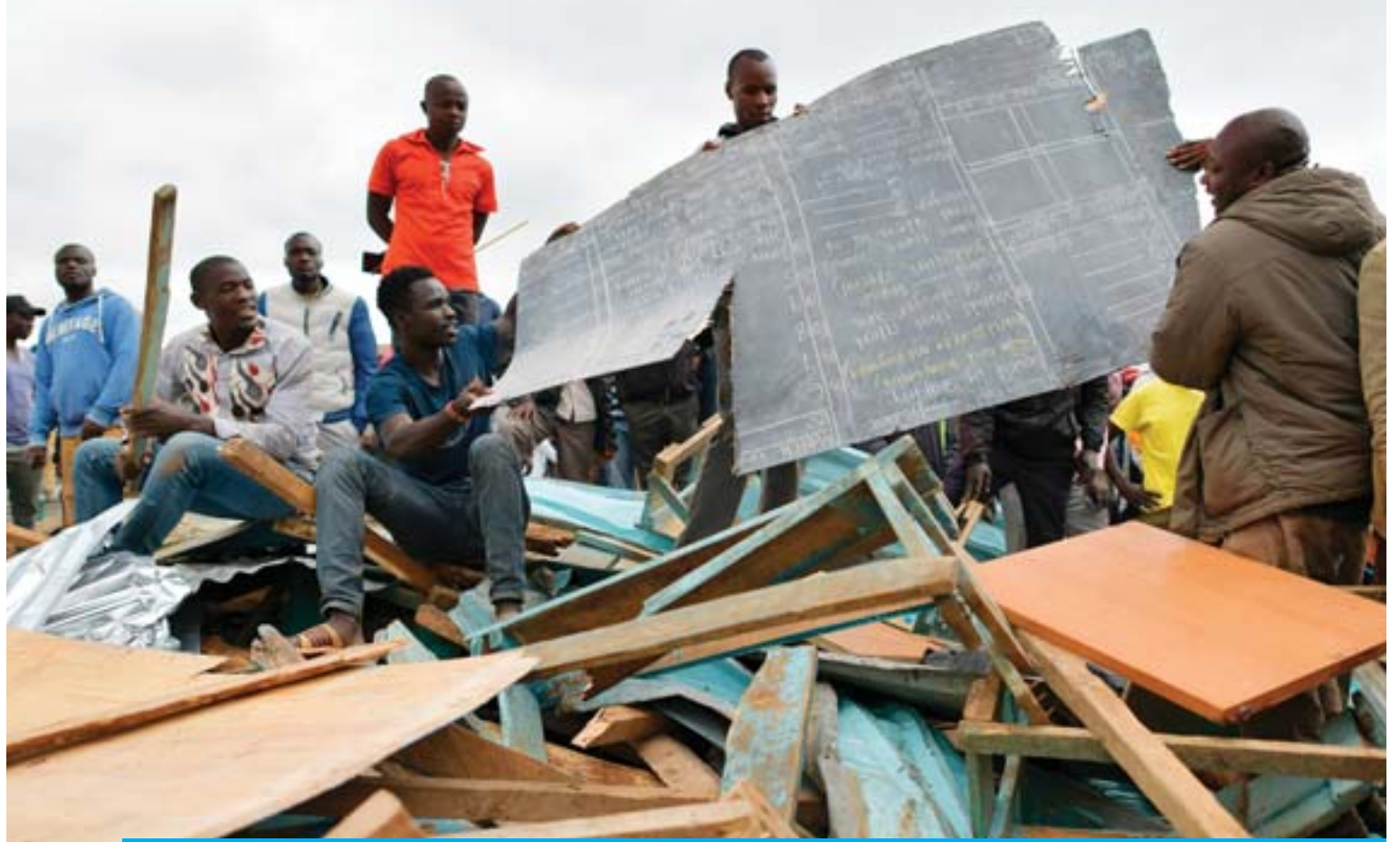
NAIROBI: People stand on debris where a classroom block collapsed at Precious Talents primary school in Nairobi's Dagoretti constituency yesterday. — AFP
