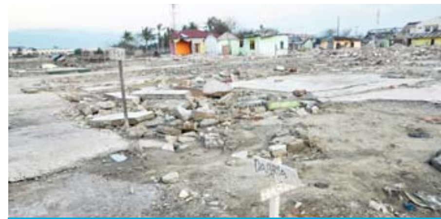
PALU, Indonesia: The remains of buildings are seen on a neighborhood area affected by liquefaction a process where the ground starts behaving like a liquid due to the September 28, 2018 earthquake, in Palu. — AFP
