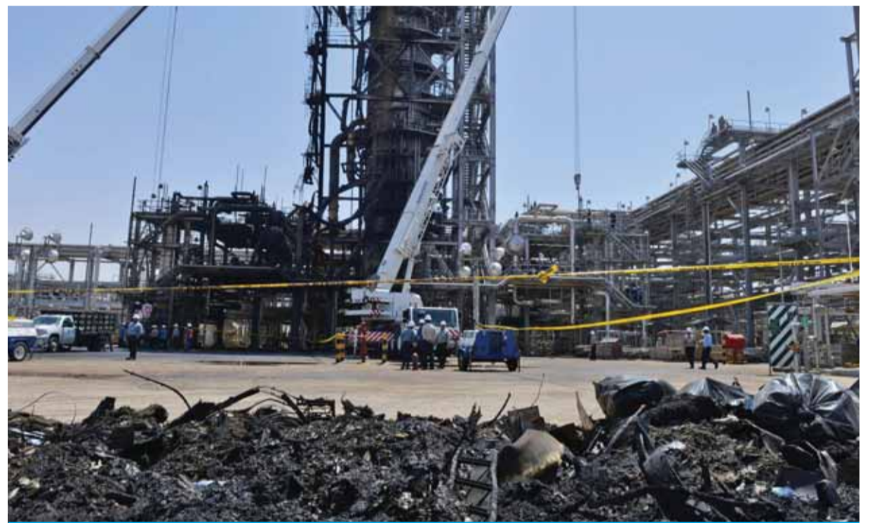
KHURAIS, Saudi Arabia: A destroyed installation in Saudi Arabia's Khurais oil processing plant is pictured on Friday. — AFP
