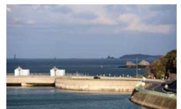
LA RICHARDAIS: Photo shows the external part of the La Rance tidal-turbine power plant in La Richardais, western France. France dreams of harnessing the energy of the oceans, from tides to currents and waves, to produce sustainable electricity. —AFP
