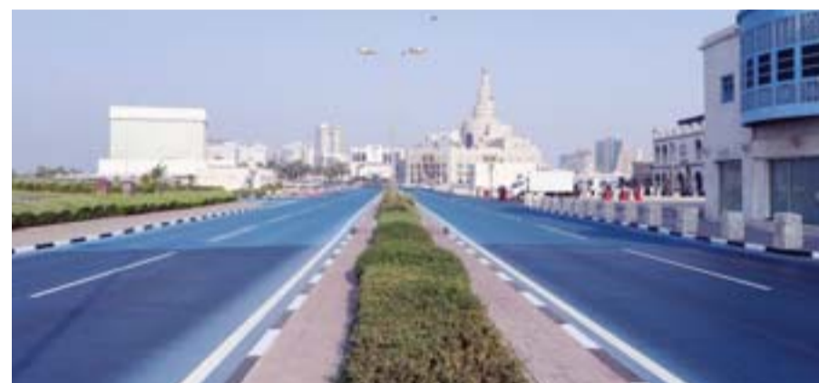
DOHA: A busy stretch of road is painted bright blue as part of an experiment to cool the tarmac surface. — AFP
