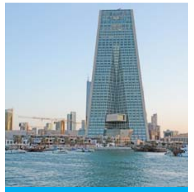
The Central Bank of Kuwait building
