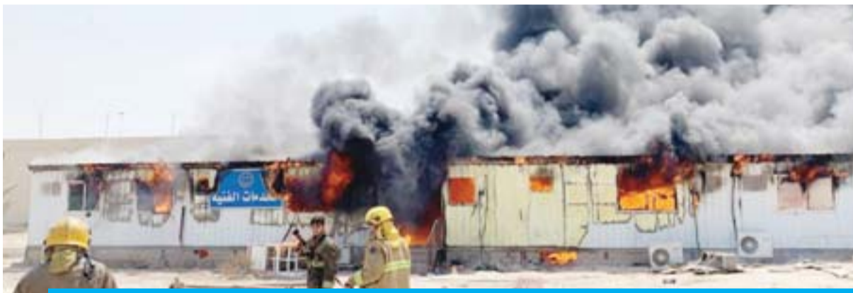
KUWAIT: Smoke billows out of a fire in makeshift homes used in the Sheikh Sabah Al-Ahmad Olympic Shooting Complex.
