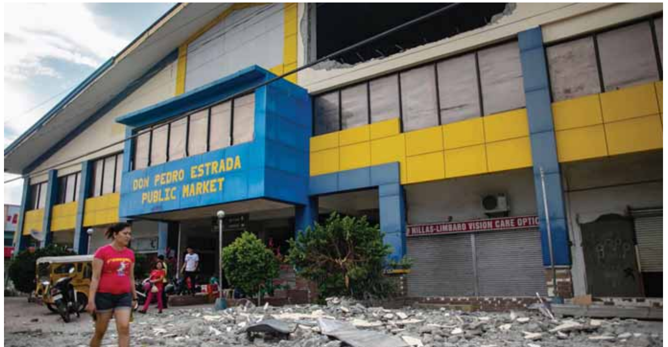
DIGOS, Philippines: A resident walks past debris from a partially damaged building after a 6.4 magnitude earthquake hit the night before in the city of Digos, Davao del Sur province on the southern Philippine island of Mindanao. —AFP
