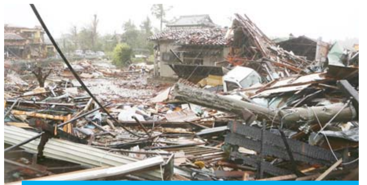
ICHIHARA: This general view shows damaged homes caused by strong wind brought by Typhoon Hagibis in Ichihara, Chiba prefecture yesterday. — AFP
