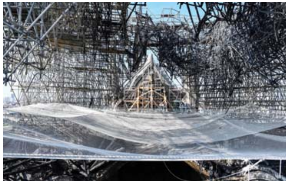
This file photo shows parts of a destroyed ribbed vault and scaffolding.
