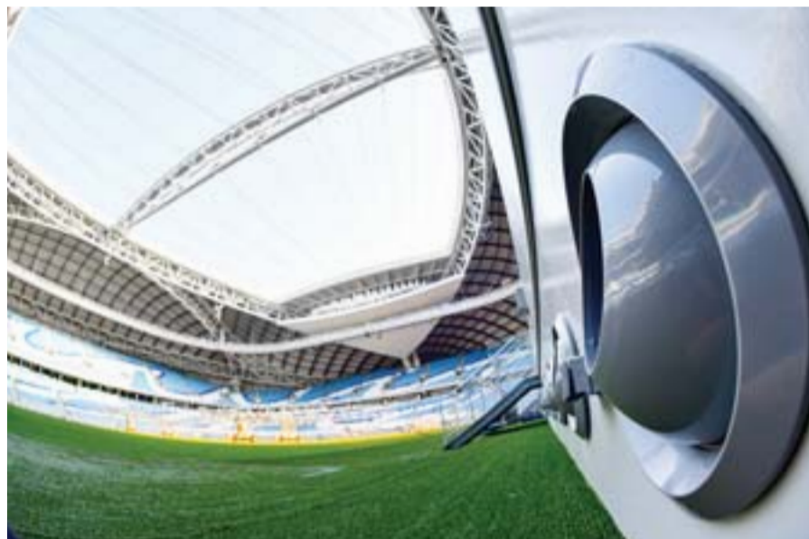
DOHA: This picture taken on September 25, 2019 shows a view of air-condition vents to be used to blow cold air at Qatar's new Al-Janoub Stadium in the capital Doha. — AFP
