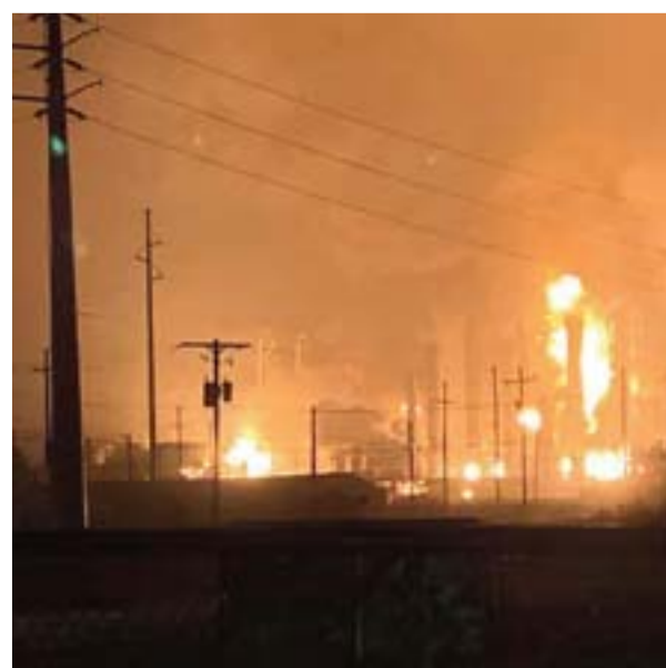
PORT NECHES, Texas: Flames are seen following an explosion at a chemical plant in this city east of Houston yesterday. — AFP
