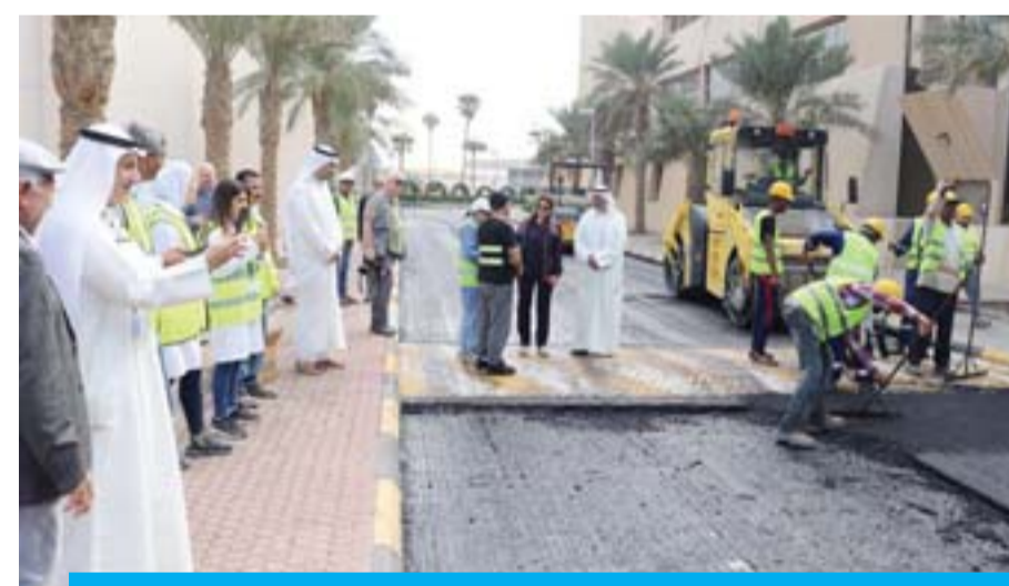
KUWAIT: Officials observe as workers pave a street with 'rubber asphalt' yesterday. — KUNA photo
