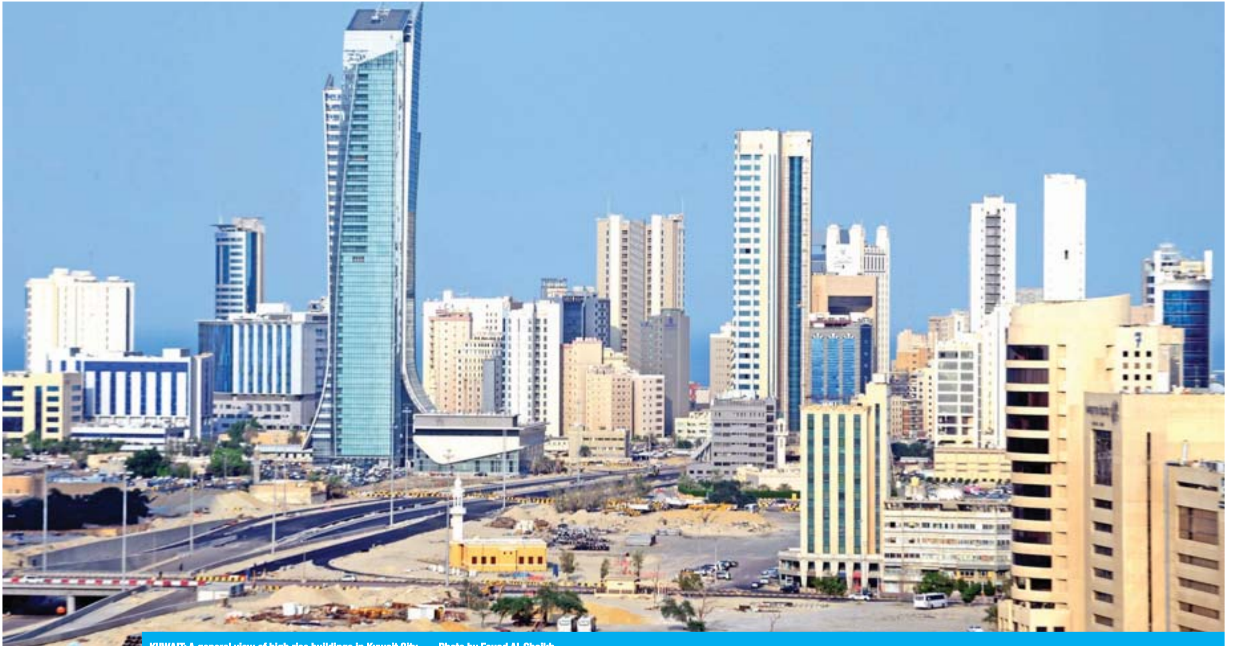
KUWAIT: A general view of high rise buildings in Kuwait City. — Photo by Fouad Al-Shalkh
